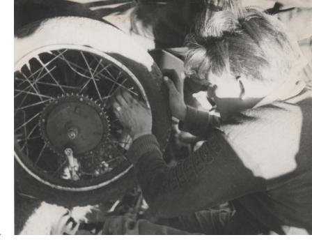
Well better before the Race than in it. Off it came and the offending clip was placed in its proper groove.
